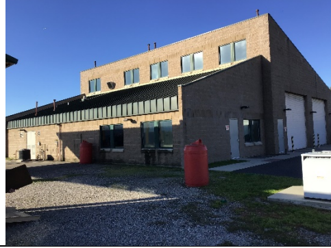
Overview- Southeast Elevation and Sector B
