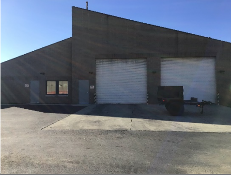
Overview- East Elevation
