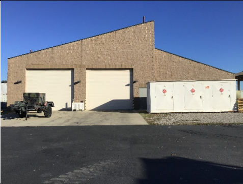
Overview- West Elevation
