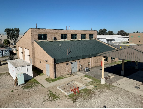
Overview- South Elevation & Sector B
