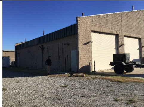
Overview- Southwest Elevation
