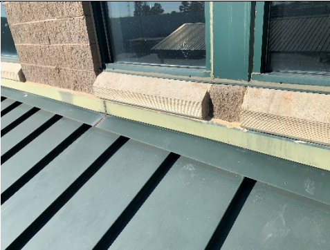
Roof to Wall- Sector B
